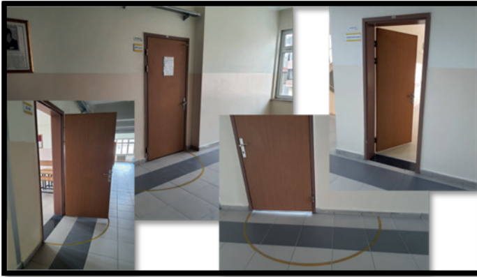
Picture 8: Door Opening Area Lines
