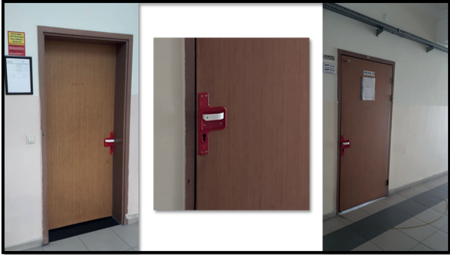
Picture 13: Door Handles Replacement
