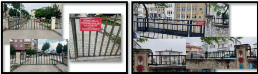
Picture 16: Garden North Side and South Side Gate
