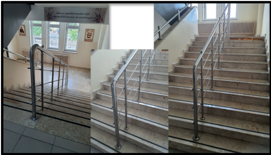
Picture 9: Handrails and Tapes
