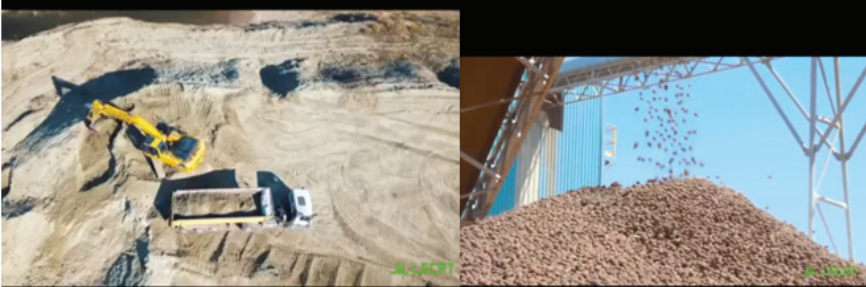
Figure 6. General view of the clay pit and the aggregate produced
