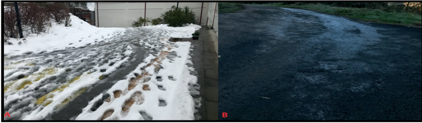
Figure 6. High-Risk Areas for Slipping on Walkways Due to Snowmelt and Refreezing of Melted Snow Water
