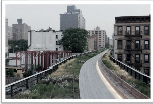
Figure 5. The High Line Park is between West 28th and 29th Streets. Photo © Iwan Baan, 2011 Source: https://placesjournal.org/article/above-grade-on-the-high-line/
