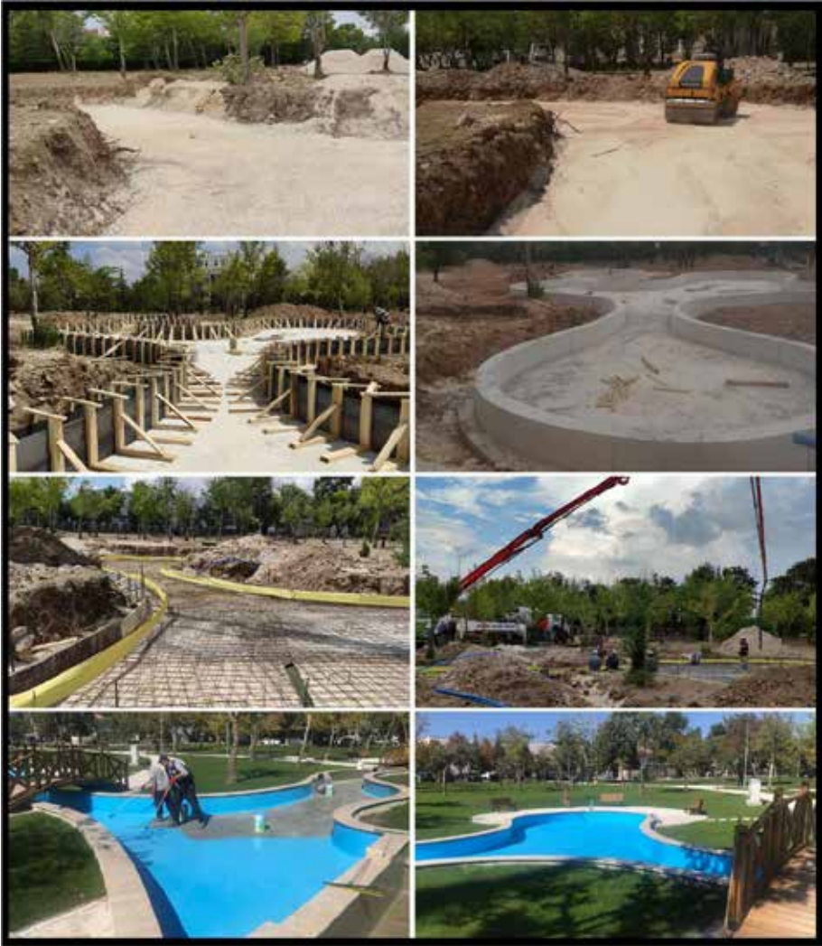
Figure 14. Ornamental Pool Implementation Phases
