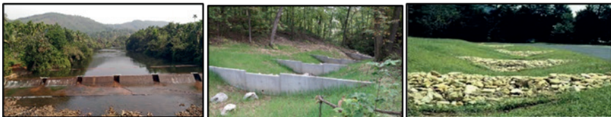
Figure 9. Check dams systems
