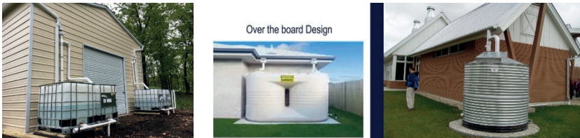
Figure 6. Rooftop collection systems
