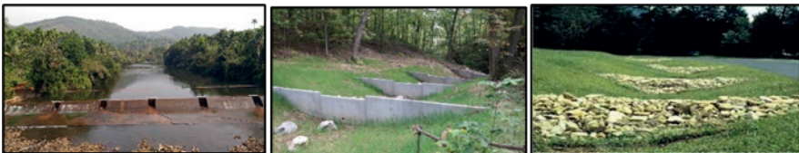
Figure 9. Check dams systems
