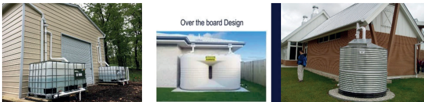
Figure 6. Rooftop collection systems
